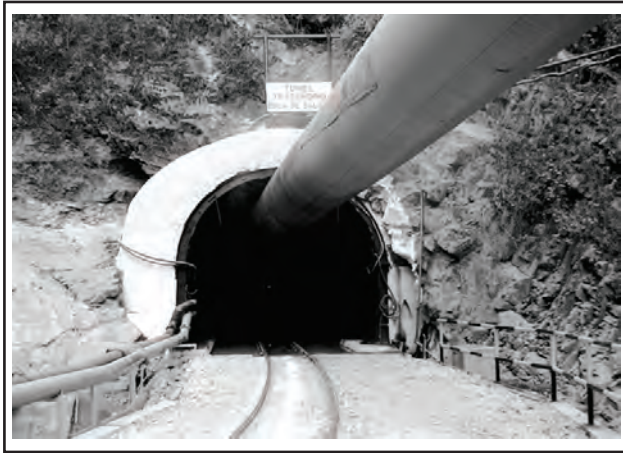
Fig. 6. An Almost Ready Tunnel Entrance [8]
