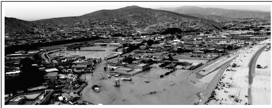
Fig.1. Areas Affected by Floods and the Destruction Caused [3]
